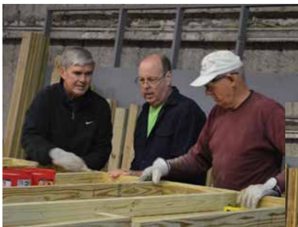
3 Volunteers Greg Morrison, Hal Hefner and Pete Mohr construct a ramp frame.
